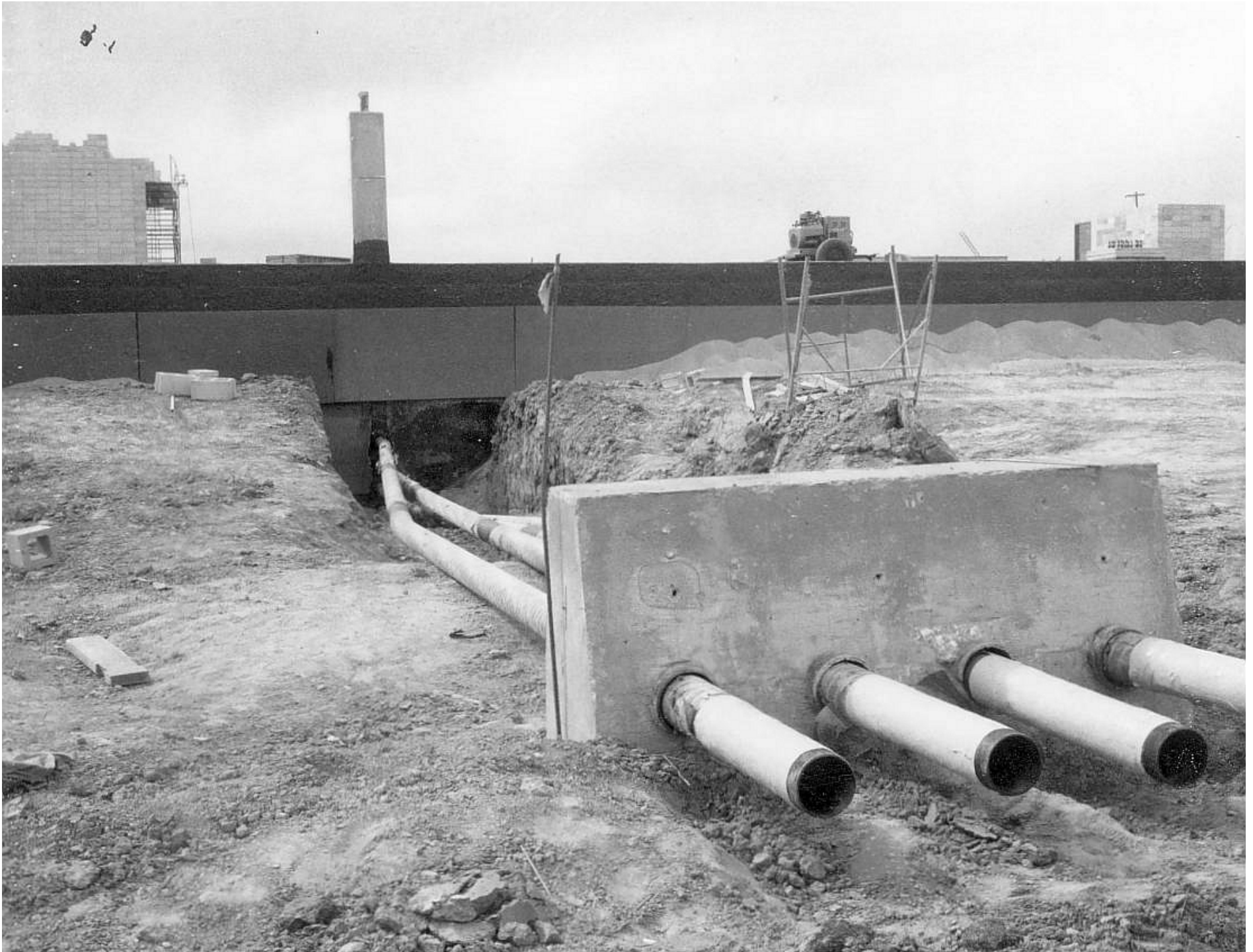
Lyons Communications Center | AUTOVON | Lyons 3-29-68 API casings _ headwall at east side of buildin
