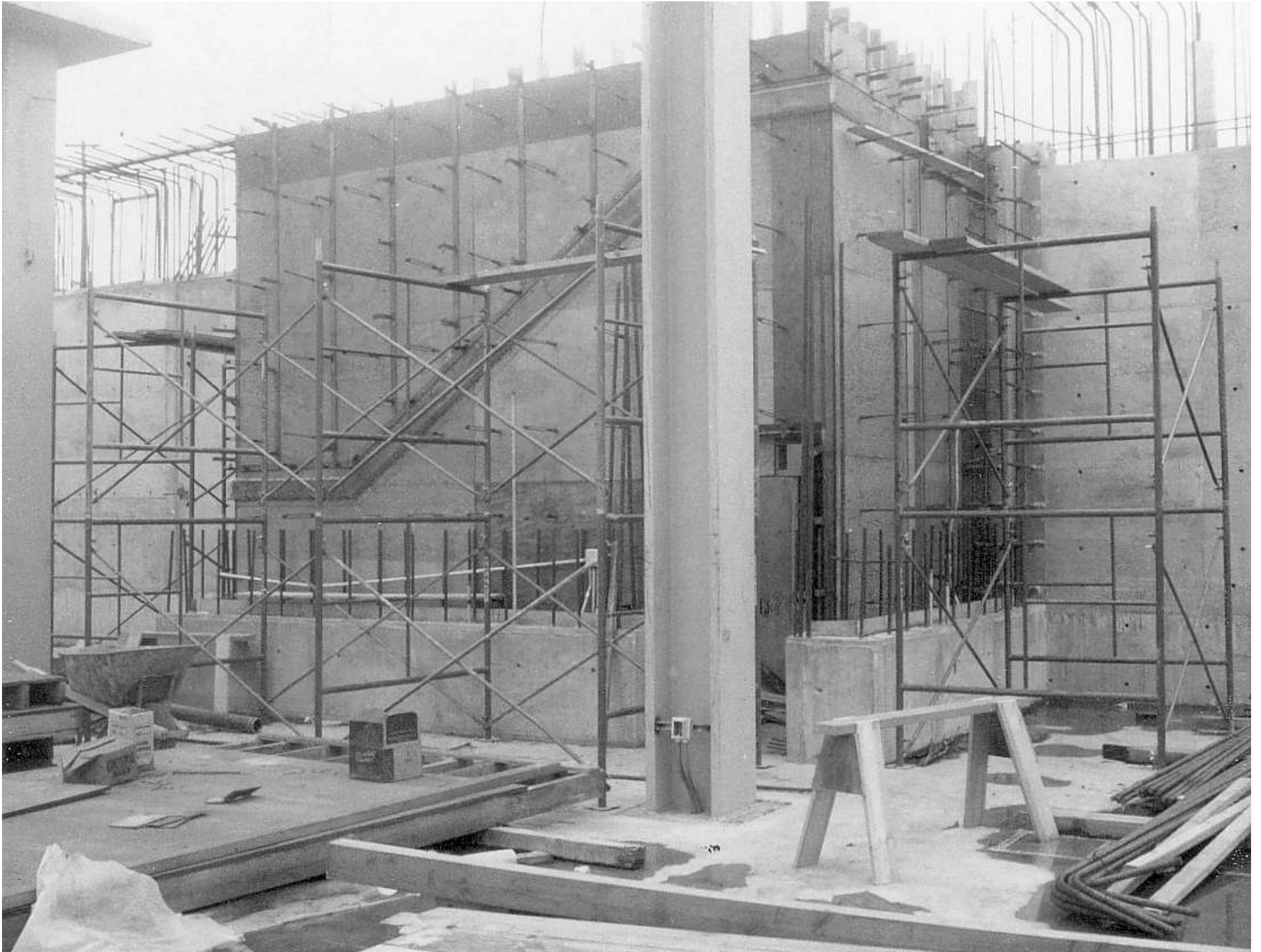
Lyons Communications Center | AUTOVON | 8-18-67 Formwork for stair #4
