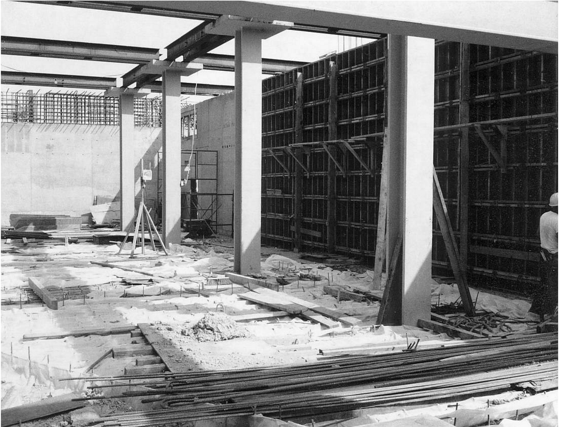
Lyons Communications Center | AUTOVON | 9-8-67 Partially completed and partially formed North wall o
