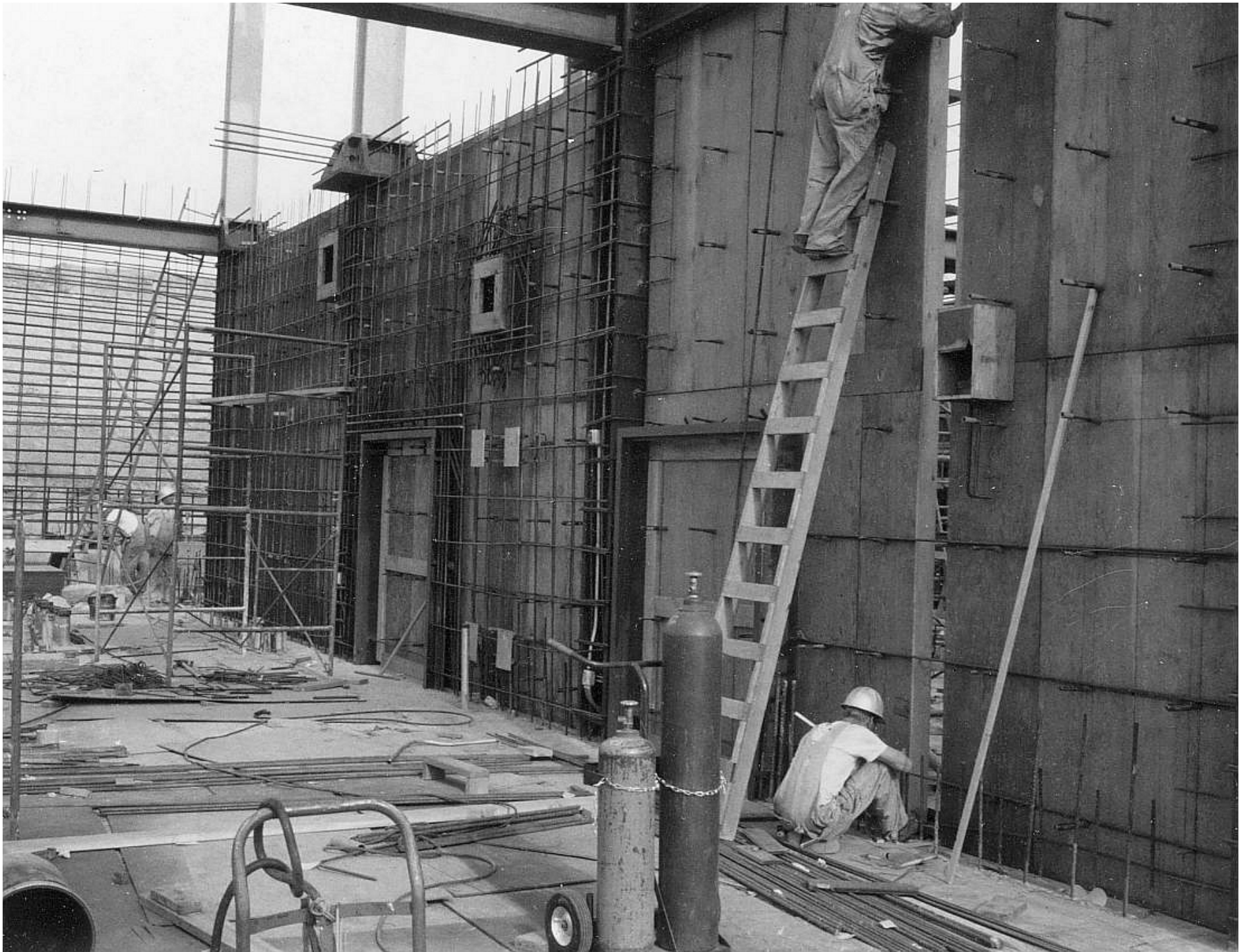
Lyons Communications Center | AUTOVON | 05-26-67 Partially formed lower wall
