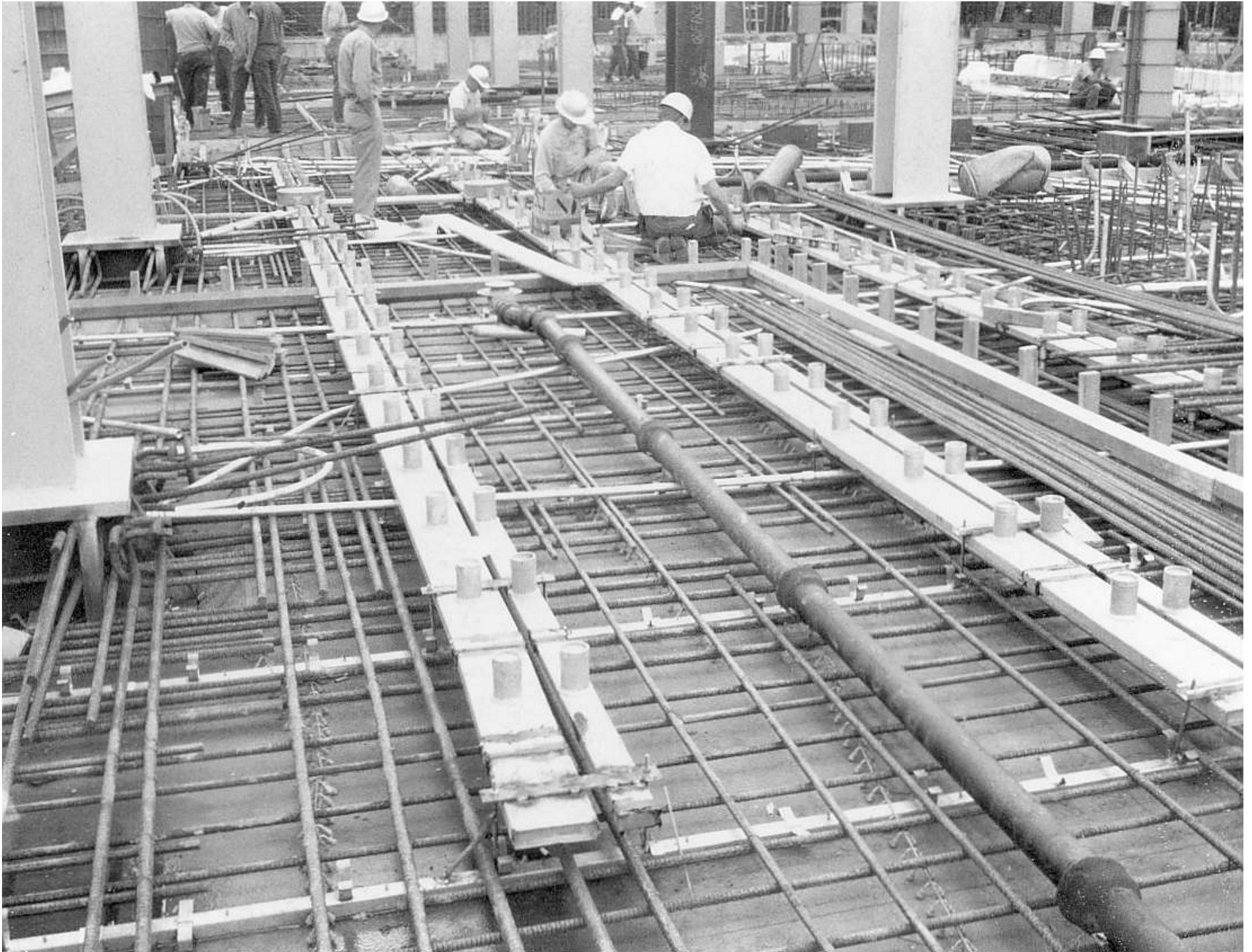
Lyons Communications Center | AUTOVON | 08-18-67 Drain piping _ underfloor duct
