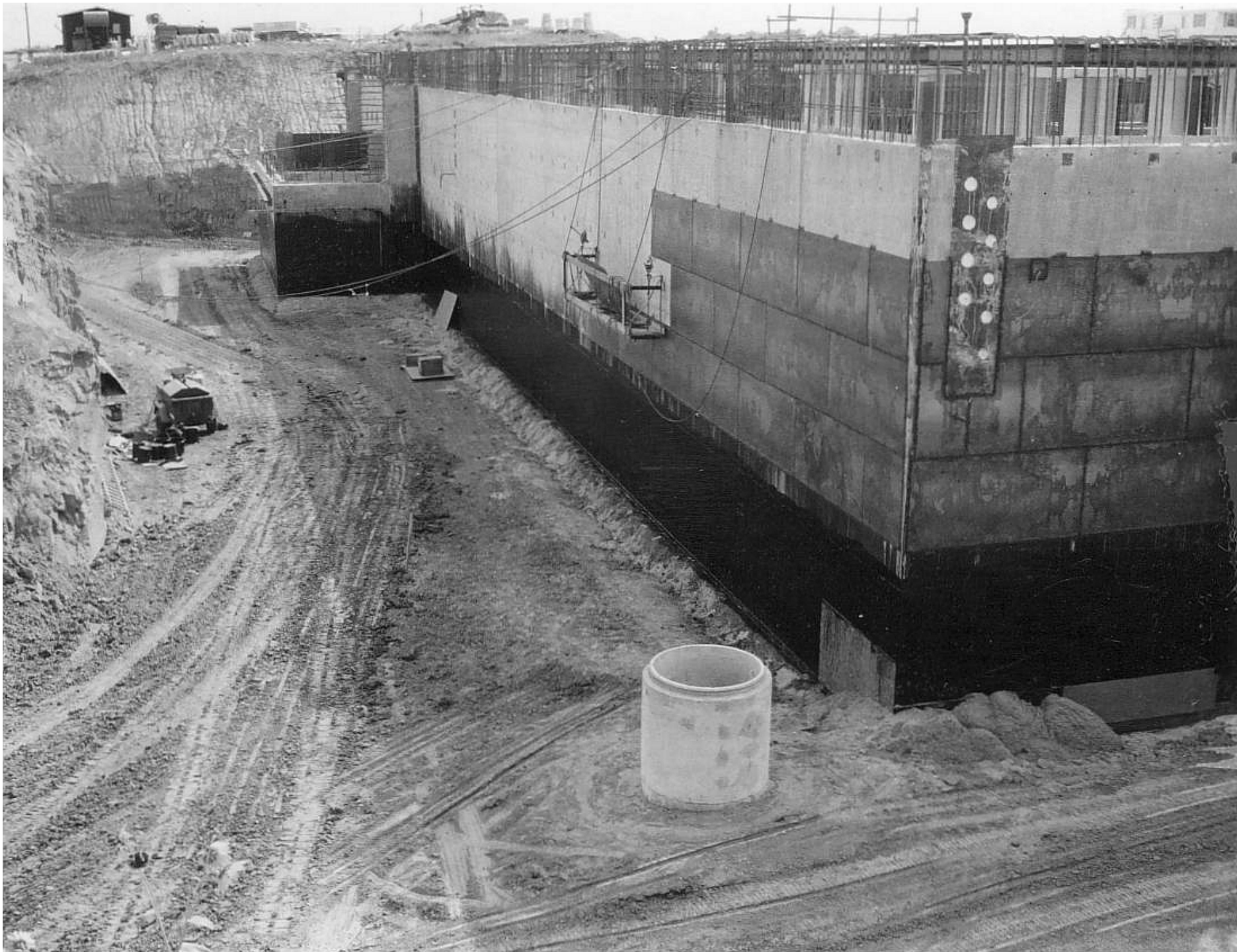
Lyons Communications Center | AUTOVON | 09-8-67 NE corner showing backfill
