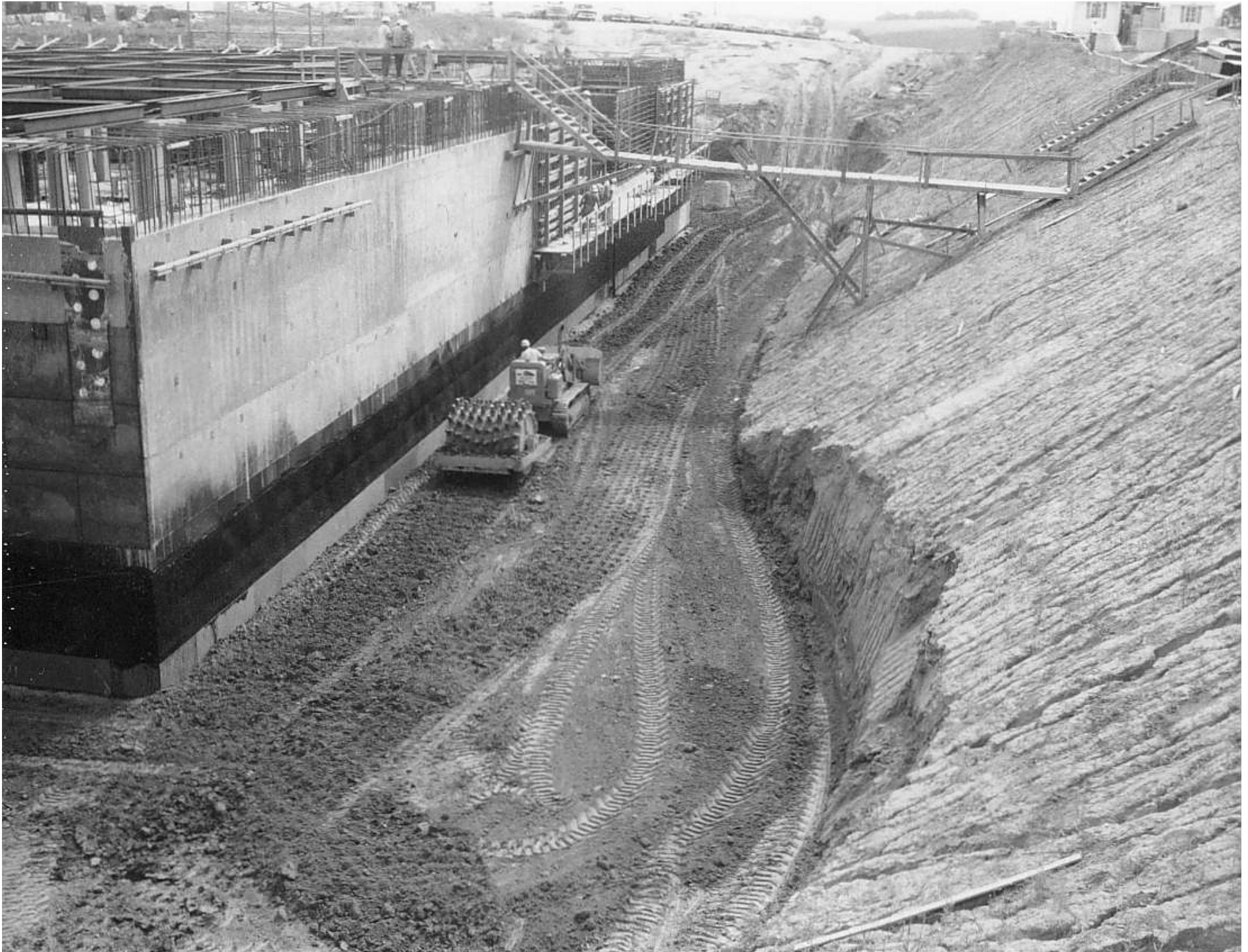
Lyons Communications Center | AUTOVON | 09-8-67 South, along West wall Backfill
