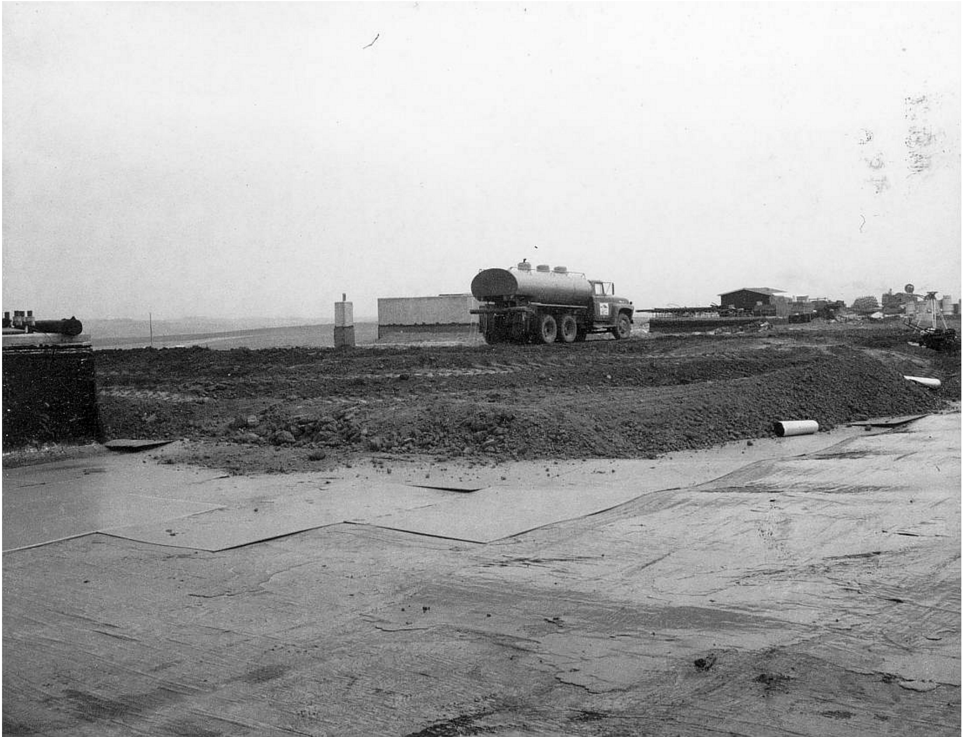
Lyons Communications Center | AUTOVON | 04-12-68 wetting down roof backfill
