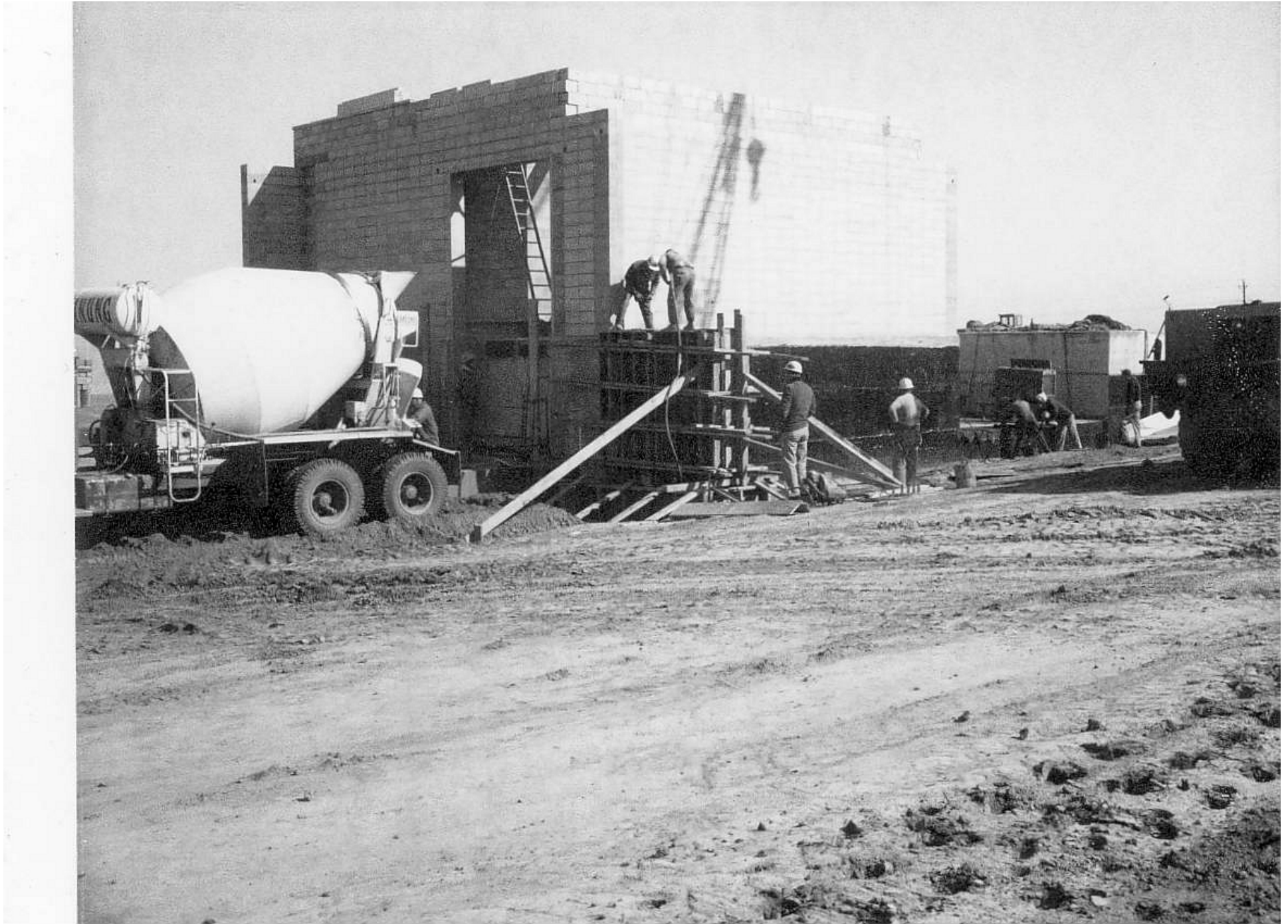
Lyons Communications Center | AUTOVON | Lyons 4-5-68 Placing concrete in retaining wall beside above
