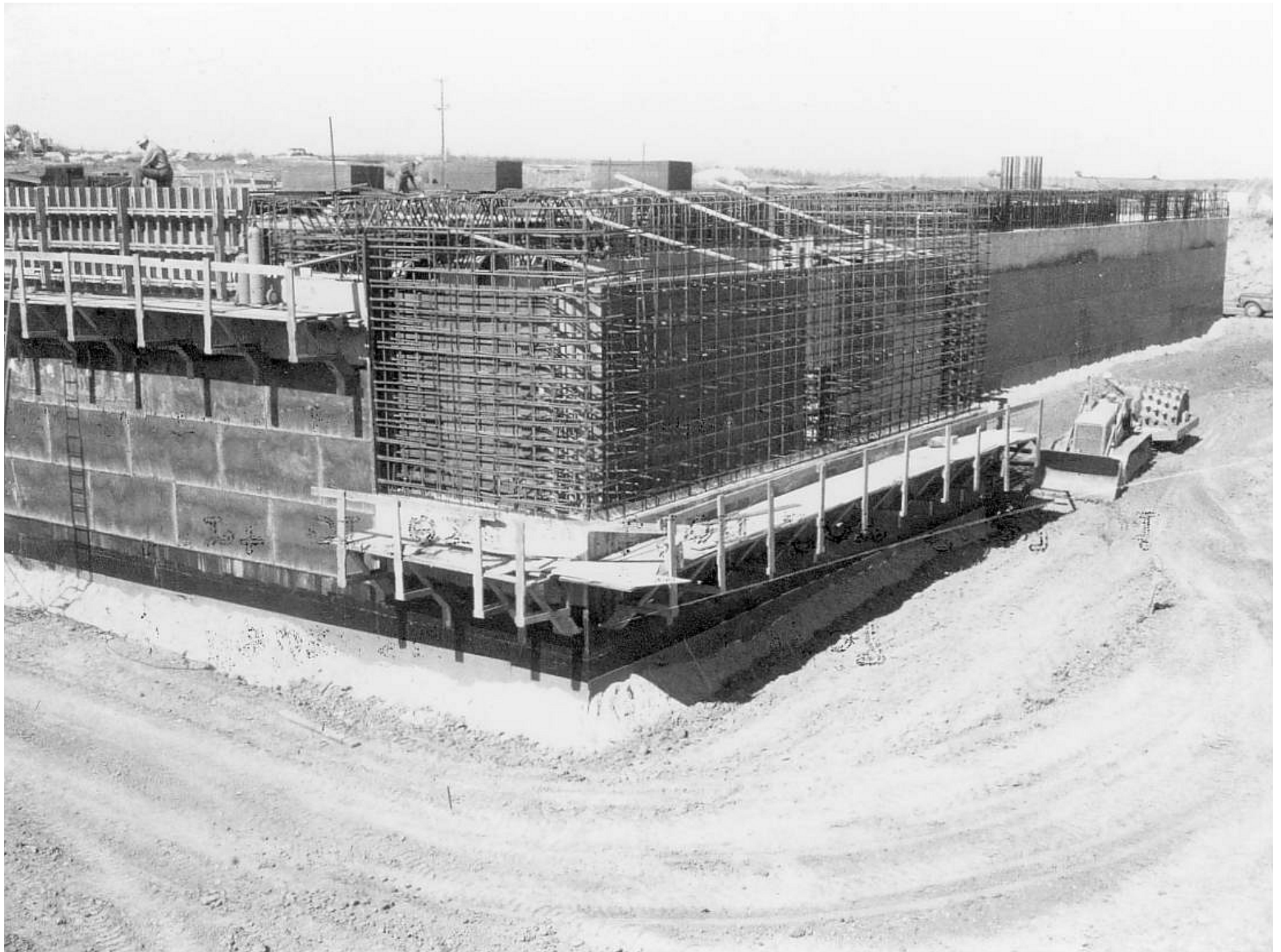
Lyons Communications Center | AUTOVON | 9-29-67 reinforcing steel at upper level walls of exhaust sh
