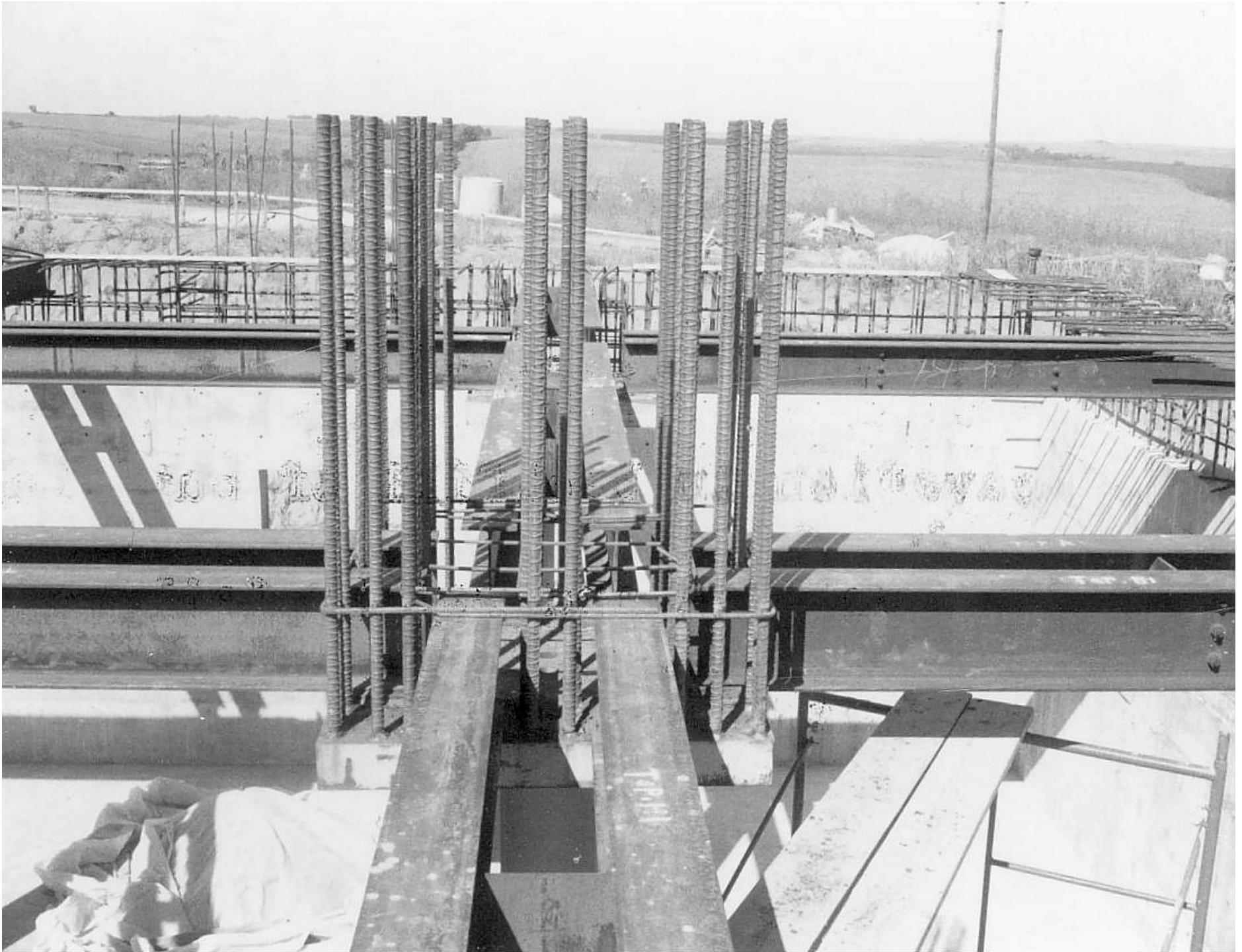
Lyons Communications Center | AUTOVON | 9-29-67 Vertical reinforcing rods welded to billet at column
