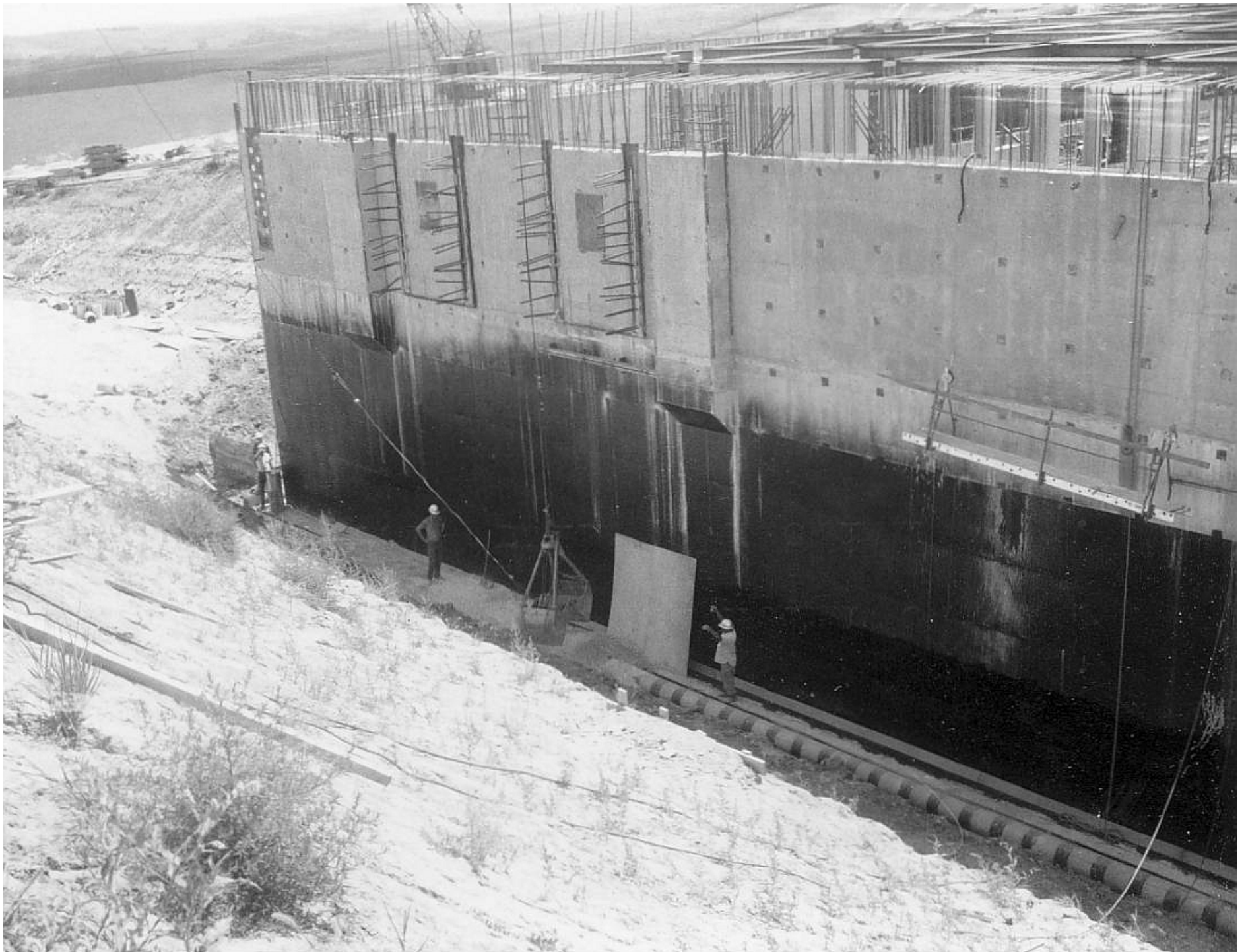
Lyons Communications Center | AUTOVON | 8-11-67 Using clam to place crushed rock over and around per
