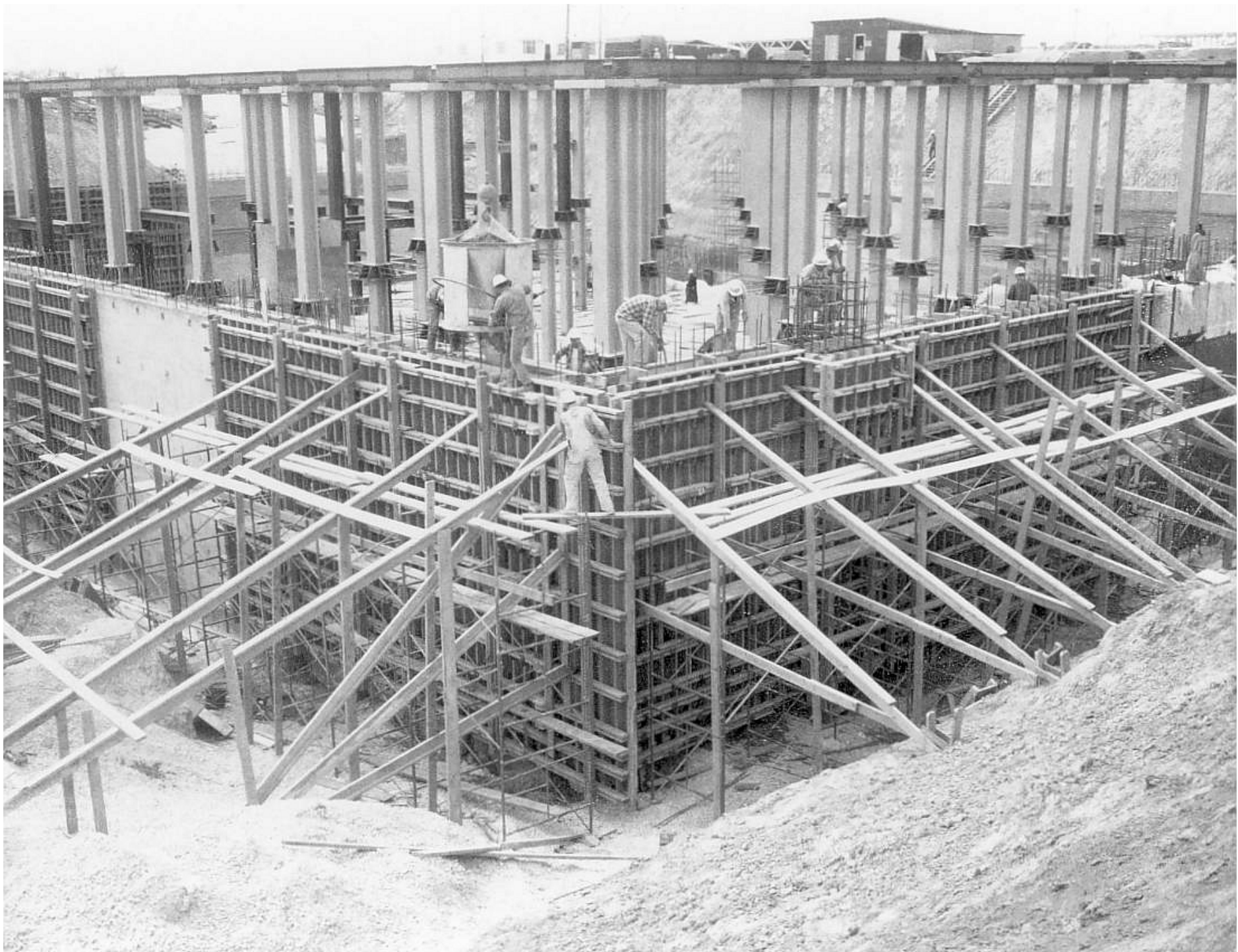
Lyons Communications Center | AUTOVON | 05-9-67 concrete in NE corner walls
