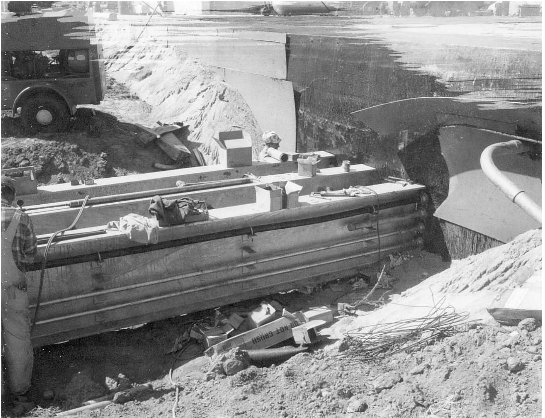
Lyons Communications Center | AUTOVON | Lyons 4-10-68 Three steel beams carrying fuel and electric s
