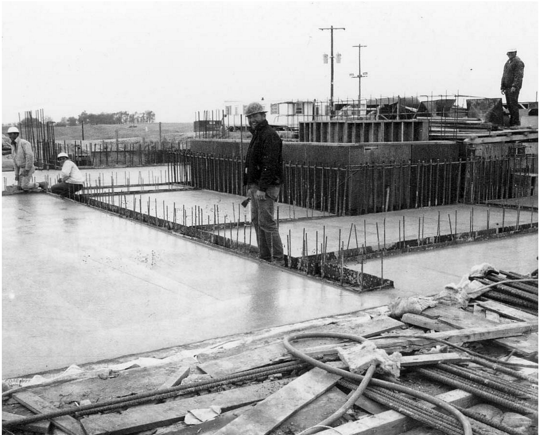
Lyons Communications Center | AUTOVON | 11-10-67 Freshly placed concrete
